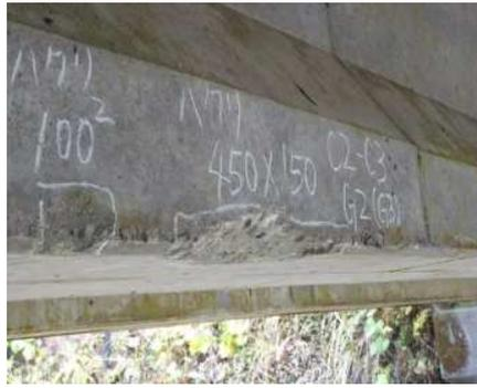
写真-主桁の欠損
